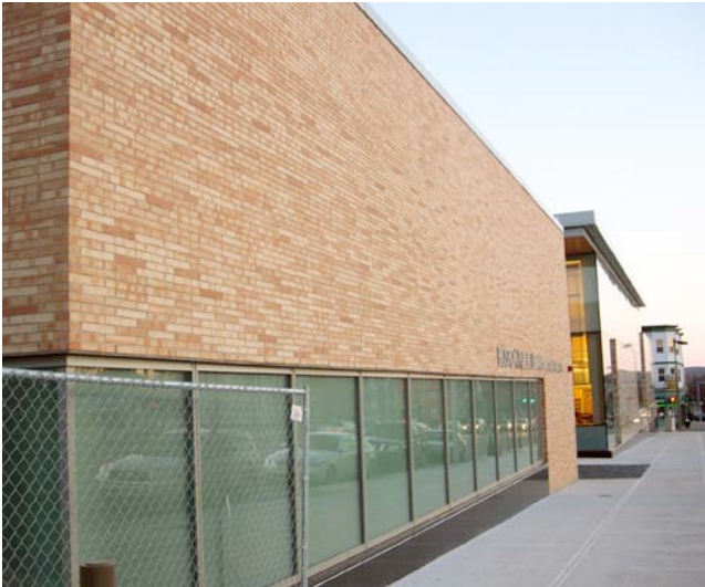
Main façade, 1350 Blue Hill Avenue
