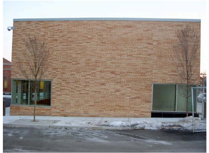
Community Room façade, parking lot entrance
