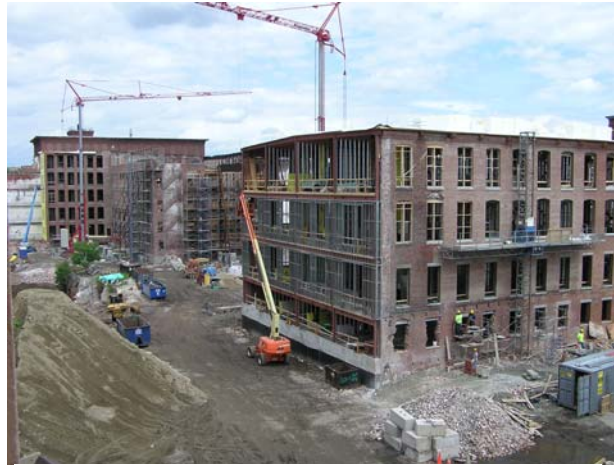
Exhibit 2 – Construction progress as of July 2010
