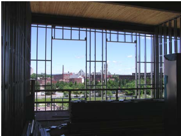
Exhibit 3 – View from inside of an apartment under construction
