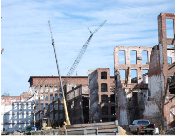
Exhibit 1 – Start of construction in late 2009
